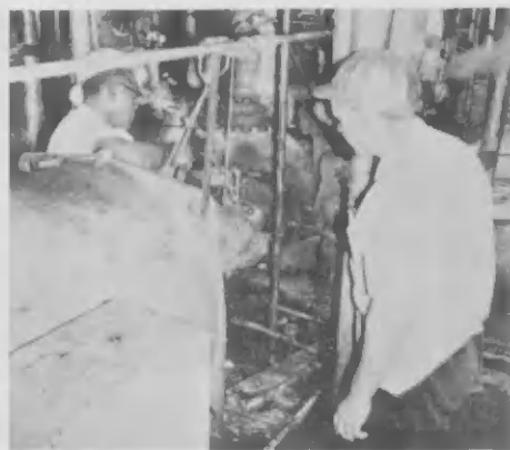
P. G. Brown (at left) performs alignment work on bottoms pump at V2AR. Super- vising the job is G. Lambrinos (TOA).
